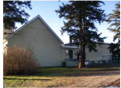
South and Rear Elevation
