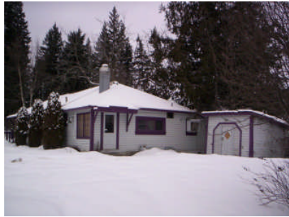
South and Rear Elevation
