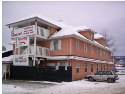
Rear and North Elevation
