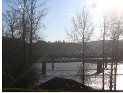
Bridge Span across Fraser River
