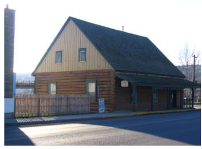
Rear and North Elevation
