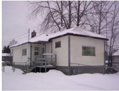
Rear and North Elevation
